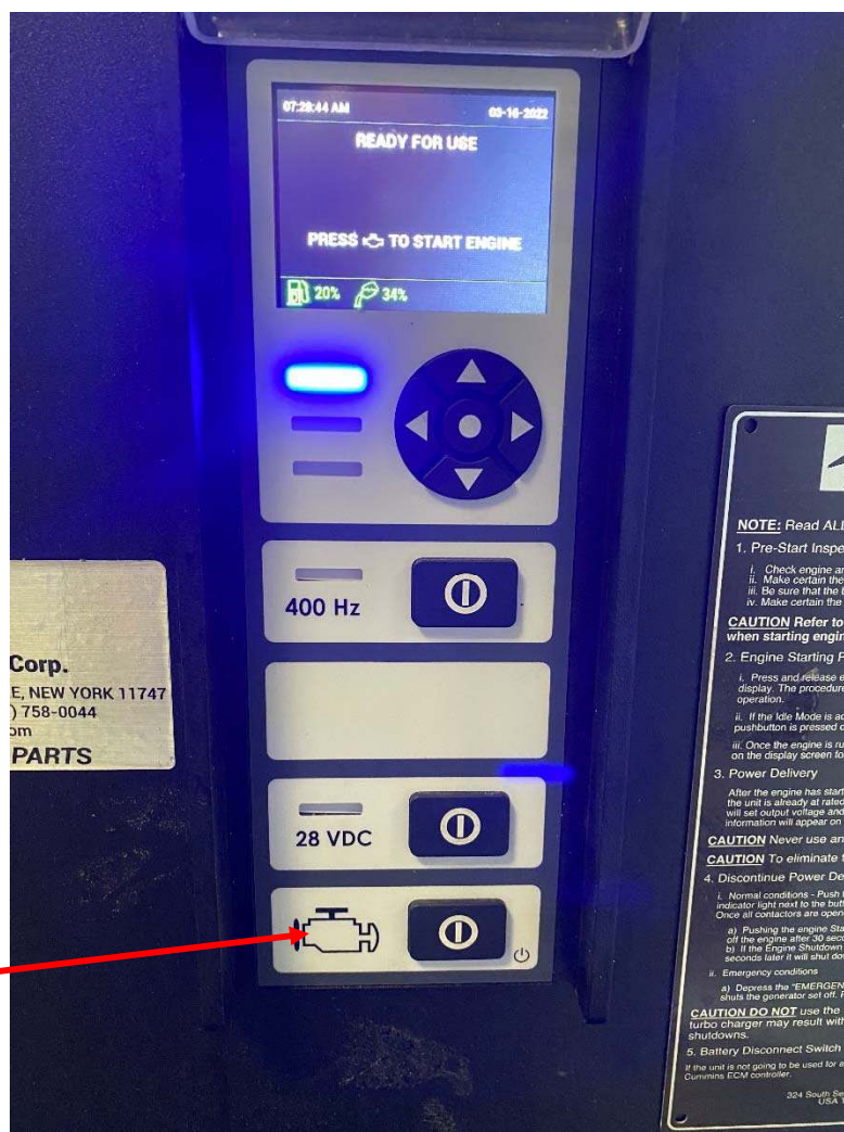
Figure 22: Press the Engine button, the ECM will now be powered.
