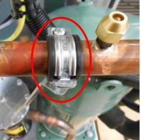
Remove insulation from condenser temperature sensor by cutting with a stanley knife. **Use caution not to cut in the wiring.** Remove temperature sensor.
